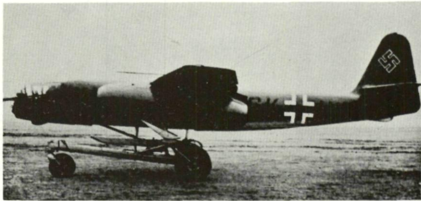
Fig. 44 The Arado 234 with skid landing gear on its trolley
