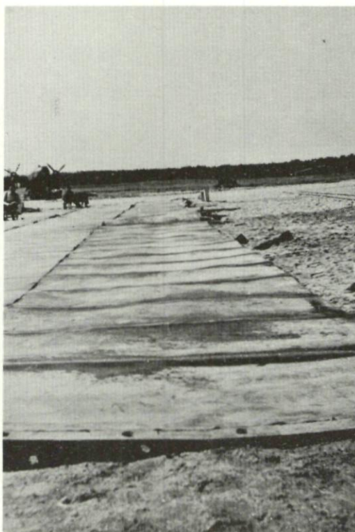
Fig. 24 Surfacing by metal sheets
