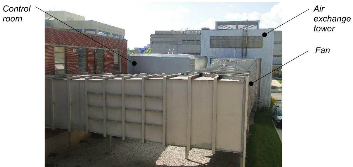
Figure 2.1-2: View of the return circuit portion of the Virginia Tech Stability Tunnel, as seen from the right hand edge of Figure 2.1-1.
